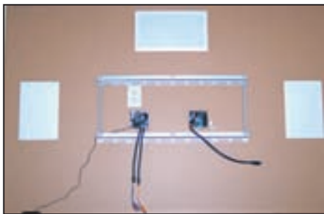
Runner cables are terminated with female connectors, eliminating the risk of fatal damage to a pin and two protective caps with pulling eyes able to withstand 30 pounds of pulling tension.
